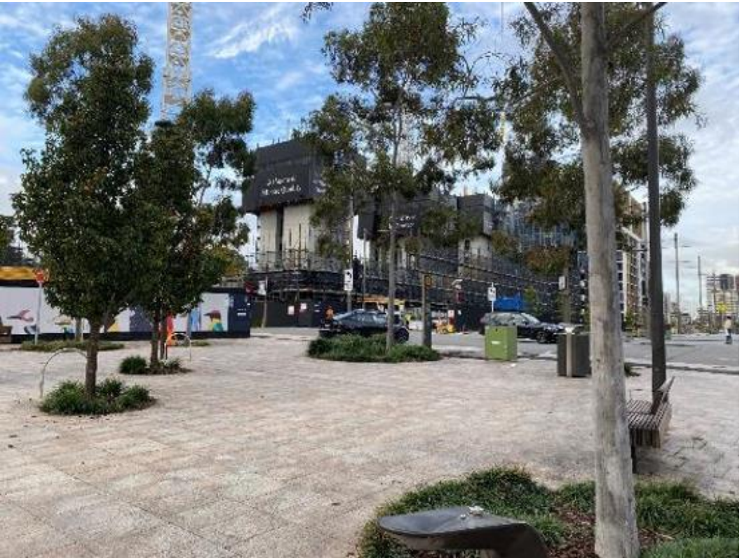
Figure 5: Site 1 looking east towards Paul Street
