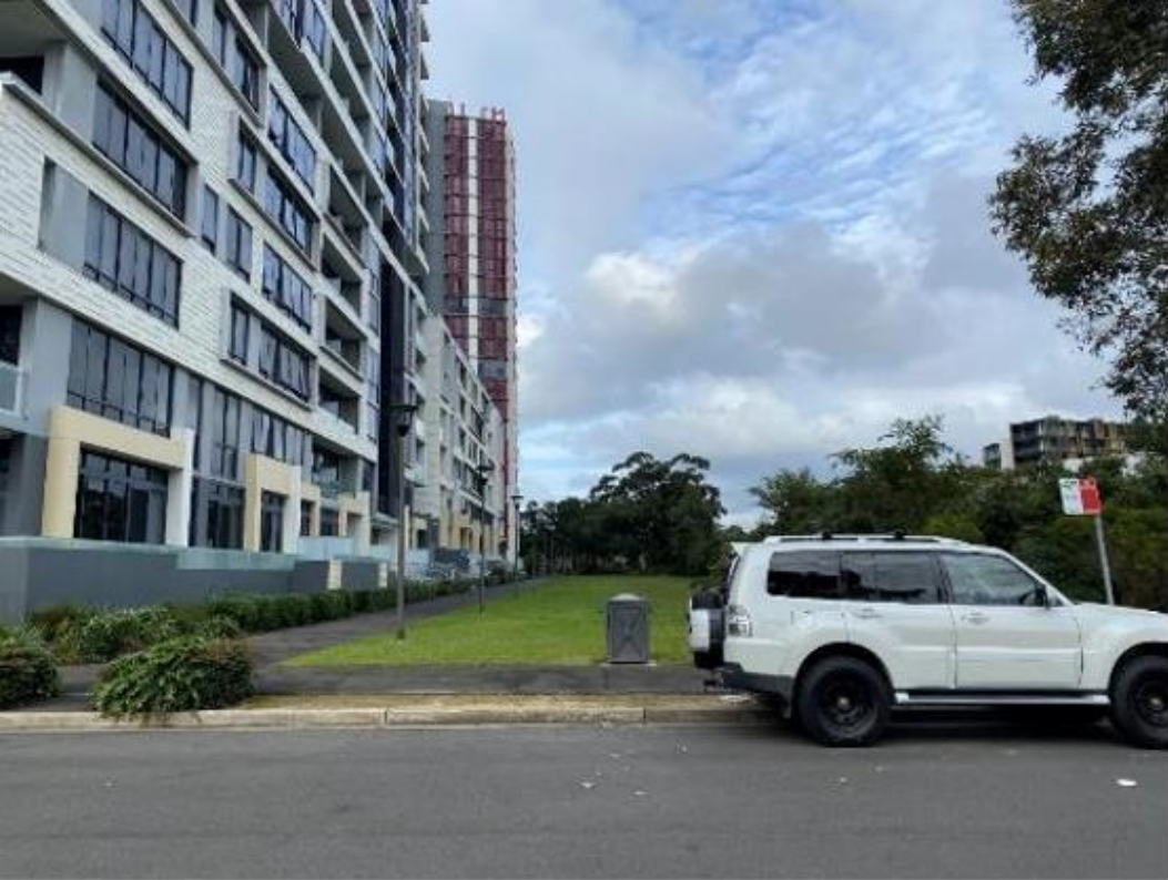
Figure 13: Site 4 viewed from Defries Avenue, looking south
